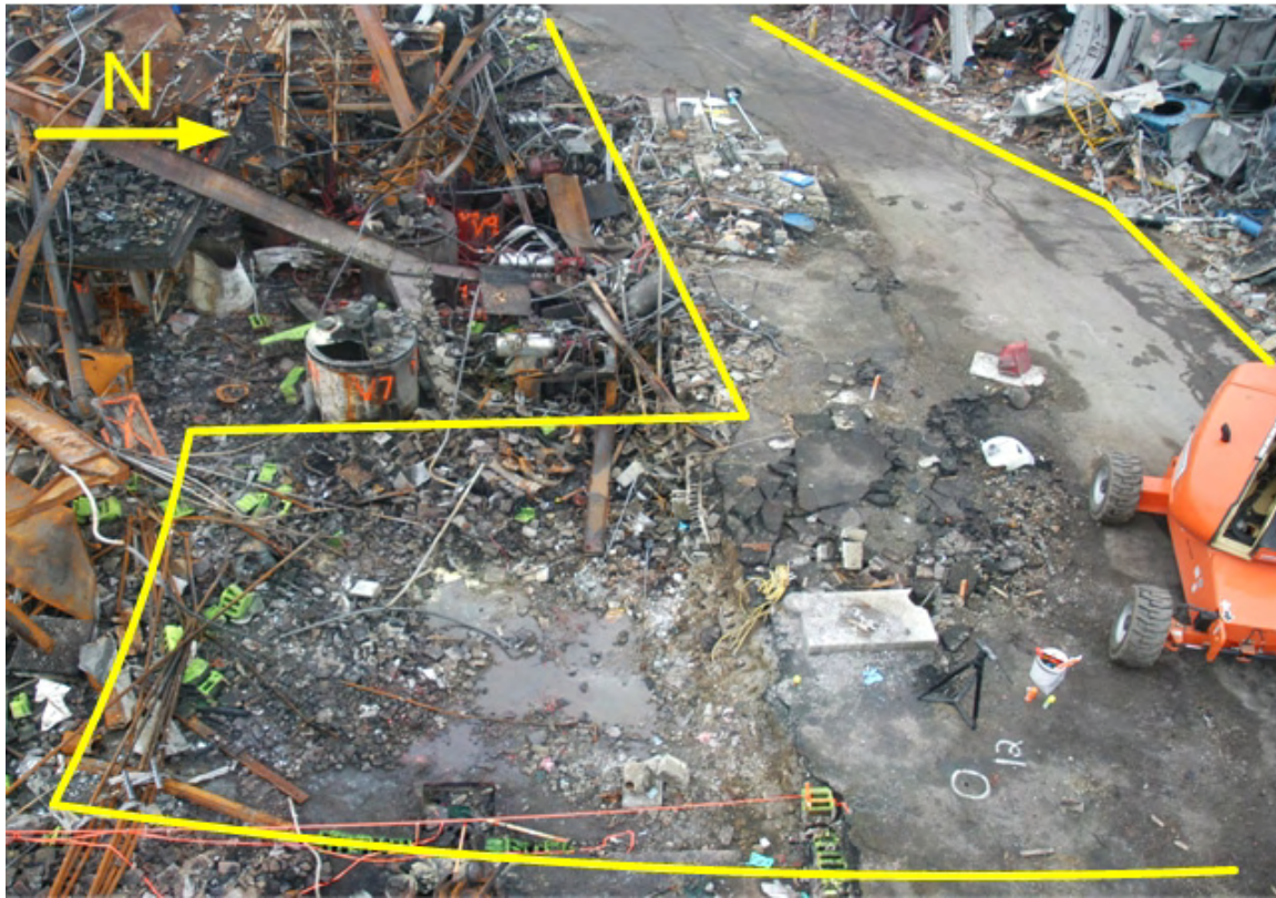
Figure 1c. Close-in photograph taken from a manlift basket on December 15, 2006, showing the extent of the evidence disturbance that occurred between November 24 and 29 (area that was cleared of debris/evidence using heavy equipment is outlined in yellow).
