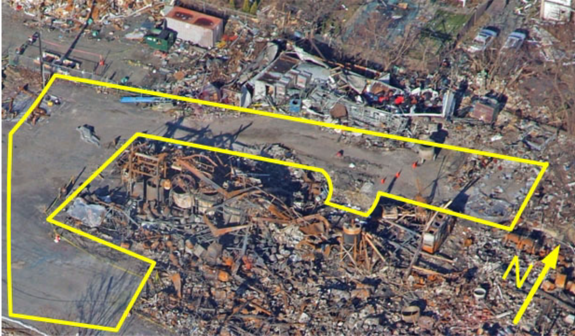
Figure 1b. Aerial photograph of Danvers, Massachusetts, explosion site taken on December 6, 2006, showing the area (outlined in yellow) that was disturbed and cleared of debris/evidence by Massachusetts fire services between November 24 and November 29, 2006.
